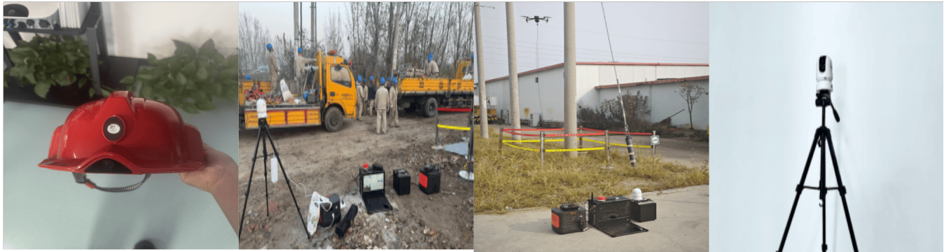
Figure 2: Deployment of multi-source image acquisition devices across heterogeneous construction sites for comprehensive visual data collection.
