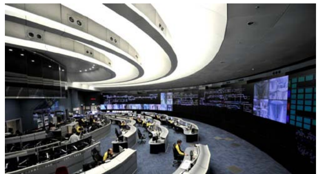
Figure 5. MTR “Super OCC” (Operations Control Center)
